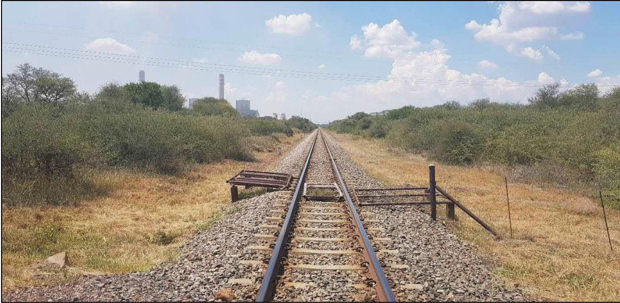
Figure 10: Railway Line between the Proposed Pipeline and SEW 2
